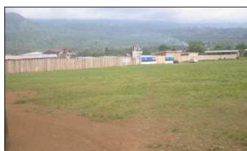
Primary schools under construction in Limbe by the Japanese
