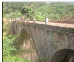
The 1911 German Ombe Bridge
